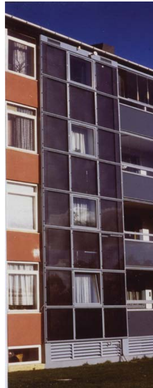
Solar panels integrated in new insulation envelope
