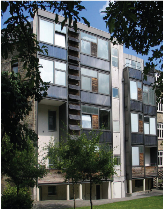
Solar panels integrated in new insulation envelope
