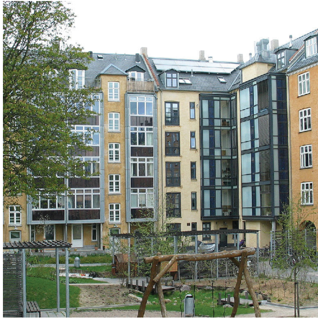
Example of after-insulation of buildings from the 1930'ties with heating panels integrated.
